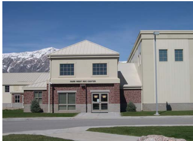
The Farr West City Recreation Center
