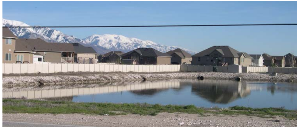
One of the City's open detention ponds
