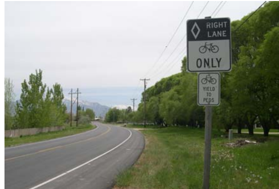
The designated bike lane along Higley Road
