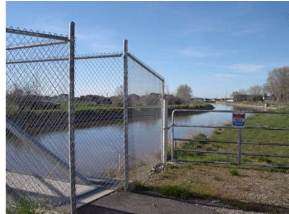
The Willard Canal at 3300 North Street
